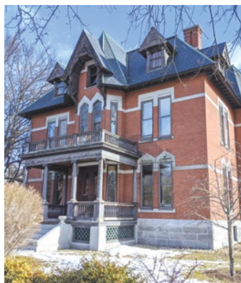
Kimball Jenkins Estate. Courtesy photos.
