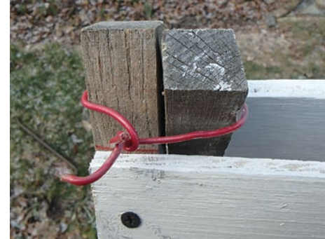
Wire the 2 sides of the A-frame together. Courtesy photo.
