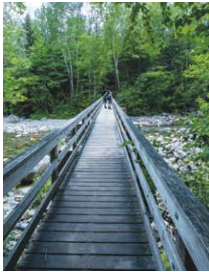
The Lincoln Woods Trail crosses Franconia Branch via a wooden footbridge.
